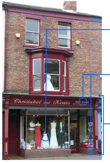
1. The window framing and its glazing should be the dominate visual element in the overall design.
