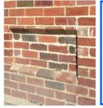
**Brick** is an alternative durable finish but designed with recessed panels incorporating a plinth, similar to a timber stall riser.
