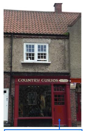
**Side located door** - allows maximum available space for a display window on narrow buildings.
