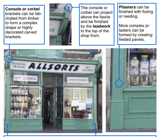
The **pilasters** can be plain boards with a plinth, (continuous with that at the stall riser), stopped by a capital mould or corbel bracket.
