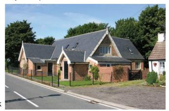
in contrasting stretcher and header bonds with a slate roof and decorative barge boards. The building consisted of a main central school hall with gabled projections to the front elevations one of which formed the entrance. Window openings consisted of stone mullioned windows with a hood mould above. A new school was opened on North Lane in 1959 replacing Elwick Hall School. The former school was left largely unused until its conversion to a house recently.
