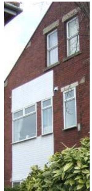
*Above: altered openings on a visible side elevation, perhaps involving removal of an original two-storey bay window. Left: clumsy PVCu detailing.*
