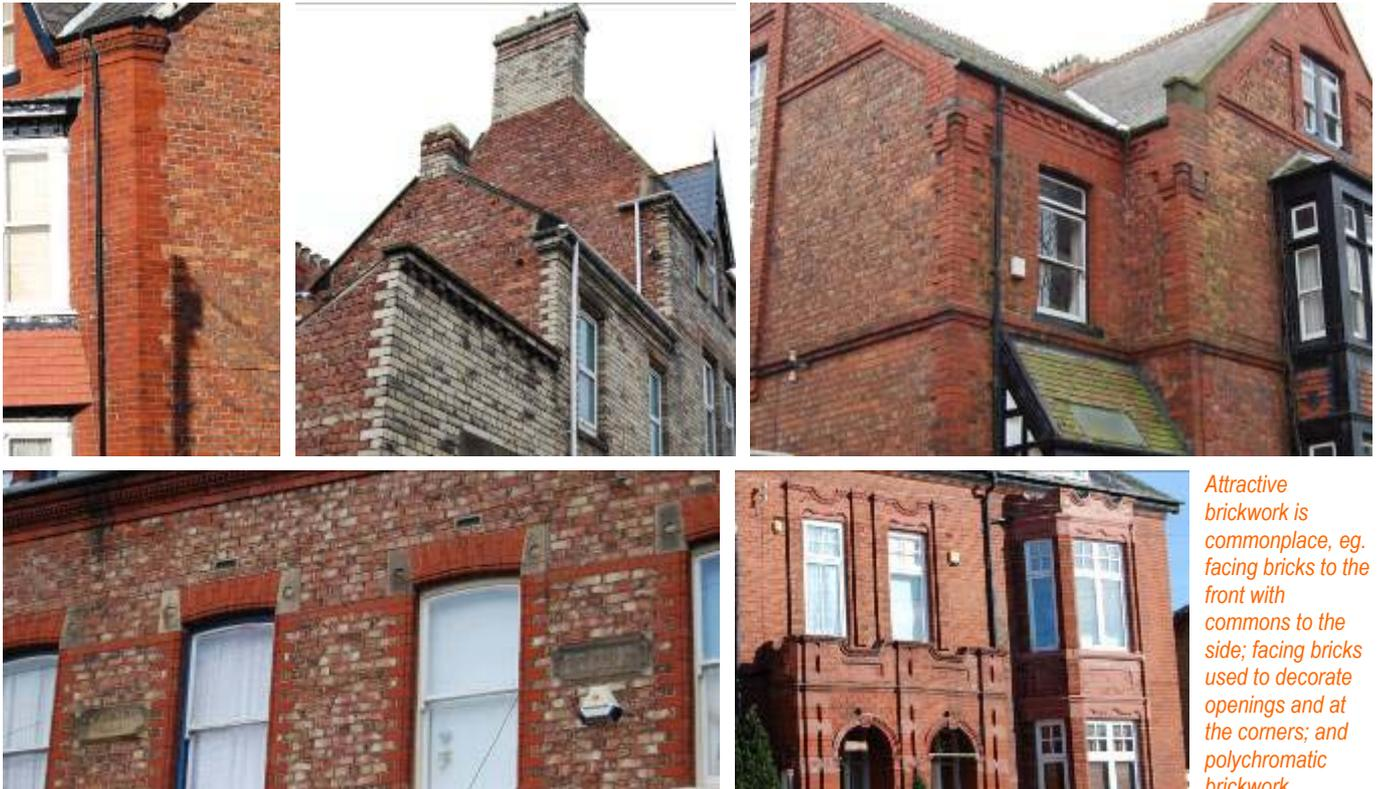
*Attractive brickwork is commonplace, eg. facing bricks to the front with commons to the side; facing bricks used to decorate openings and at the corners; and polychromatic brickwork*
