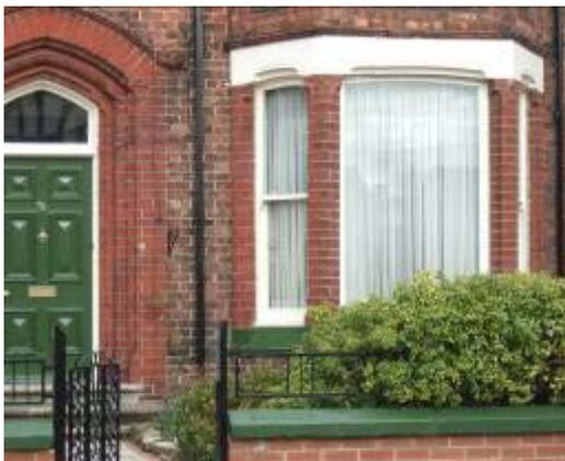
Like doorways, windows are key features in the architecture of the area used to enliven elevations. Most window openings are vertical; where they are more square or horizontal openings (notably in the later semis in the west of the area), the windows themselves are divided by mullions to create verticality. The strong verticality of windows is a key part of most of the architectural styles in the area. On Victoria Road, it balances out the width of the double-fronted buildings' forms.
