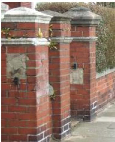
Traditionally, the low boundary walls would have been topped with low metal railings between the piers, matched by gates to the paths or drives. The earliest ones would have been in iron individually leaded into the plinths, and would have been very decorative. It is very rare for these to survive but a good stretch is in place on the side wall of No.36 Clifton Avenue, whilst several solo panels of railings survive built in to porches in many locations (notably Linden Grove).
