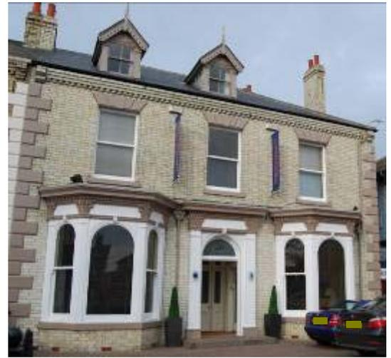
Bricks are predominantly laid in simple stretcher bond on front elevations, with English garden wall bond used mainly on side and rear elevations, with either 3 or 5 rows of stretchers to 1 of headers. Examples of Flemish bond (alternate headers and stretchers in every course, with headers placed centrally between the stretcher immediately above and below) are a rare stylish flourish, seemingly only found at St
