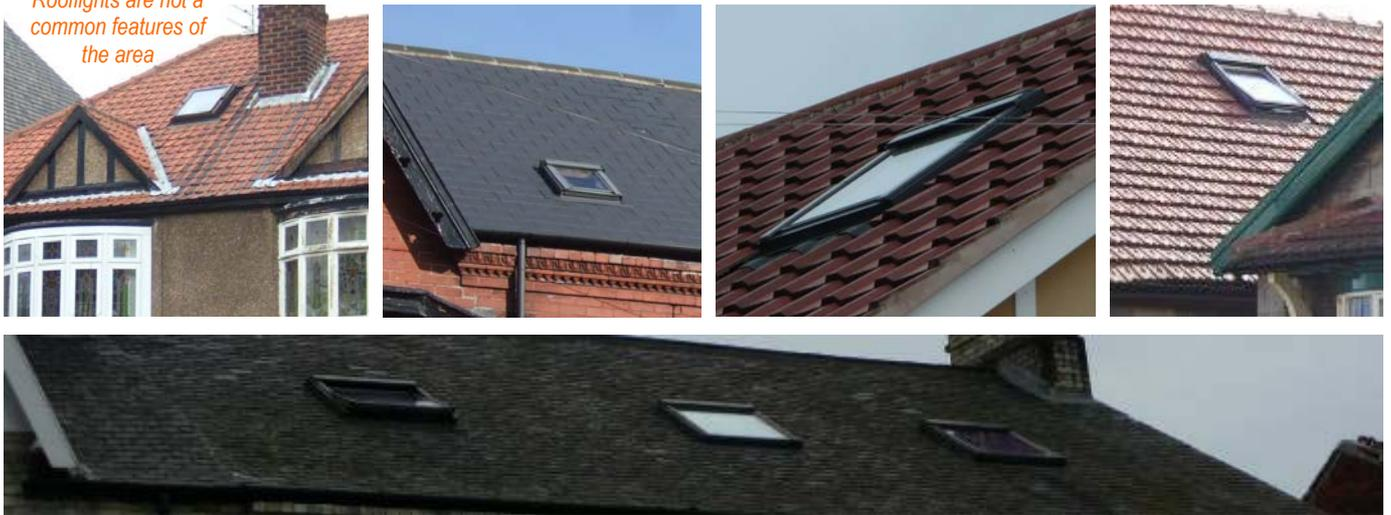
Rooflights are not a traditional feature of the area’s architecture although the odd historic one is seen, often small metal features or ‘glass slates’ (small frameless panes of glass placed in the roof). Large modern rooflights have been added to some roof slopes, some more subtle than others, but there is not a great number of them which works to protect the roofscape. Generally large modern rooflights tend to detract from historic roofscapes through their size, profile and positioning.
