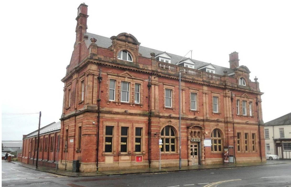
Fig 83. The former Post Office, Whitby Street.
