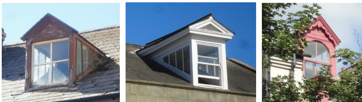
Figs 23, 24, 25. Examples of the distinctive side-glazed dormers.
