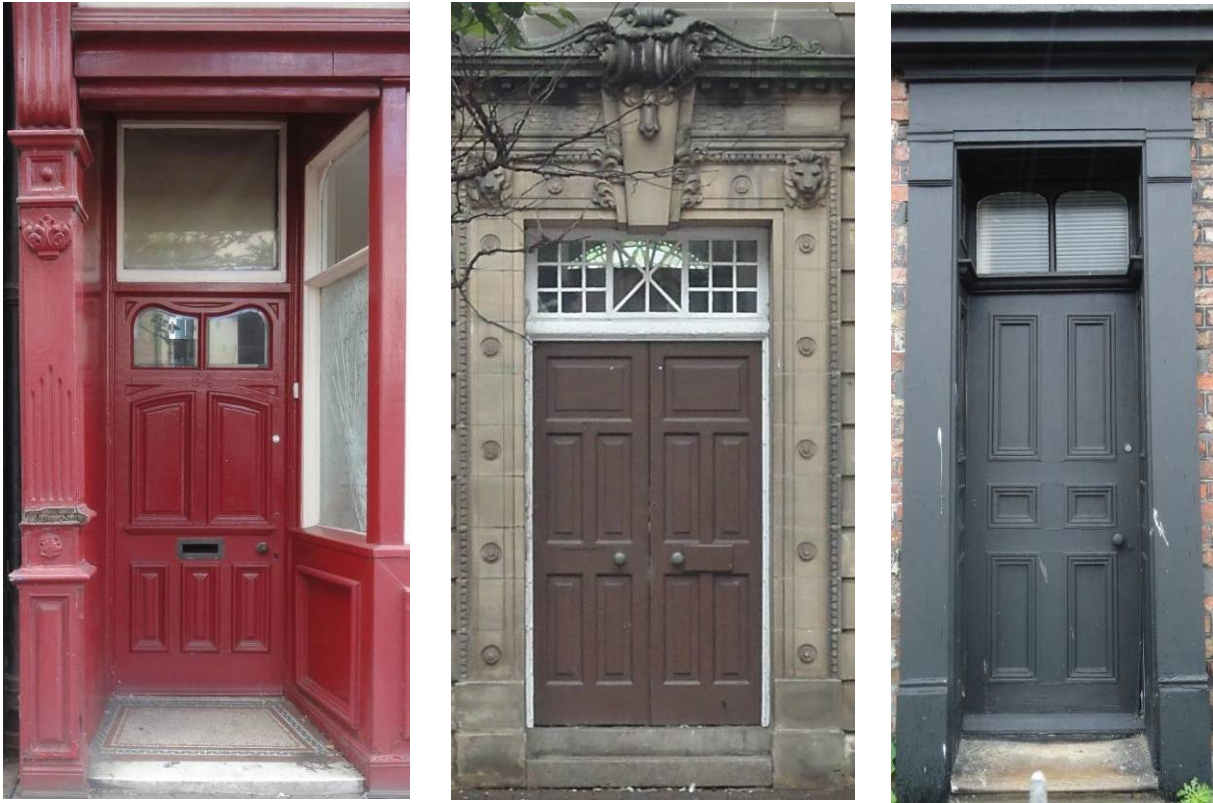
Figs 38-40. Distinctive doors, doorways and fanlights distinguish the conservation area.
