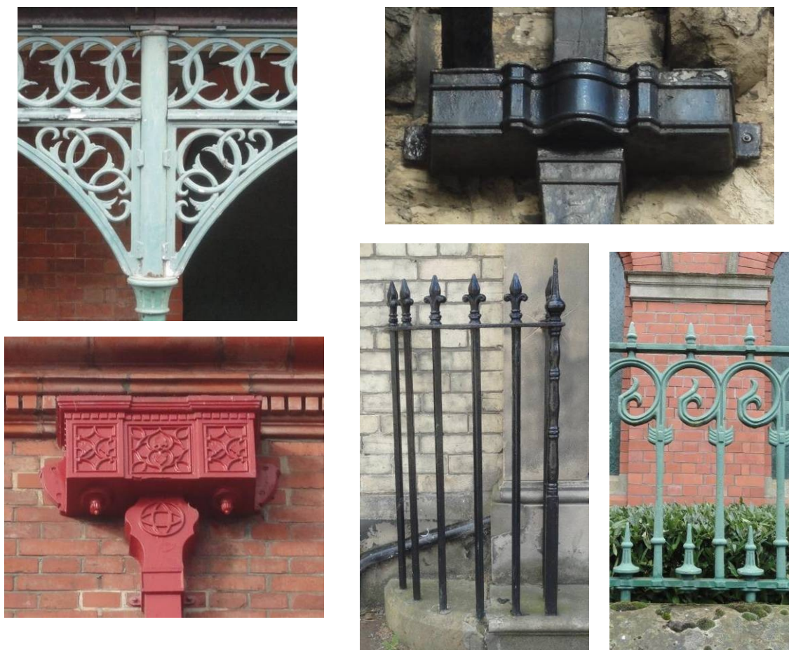
Fig 32. Examples of the fine ironwork abounding in the conservation area.
