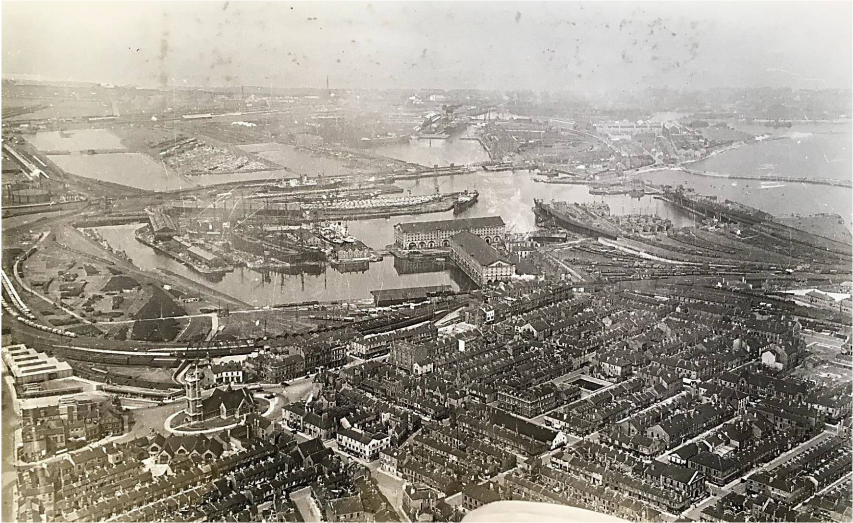
Fig 2. Aerial photograph of West Hartlepool, 1946, taken from the south.
