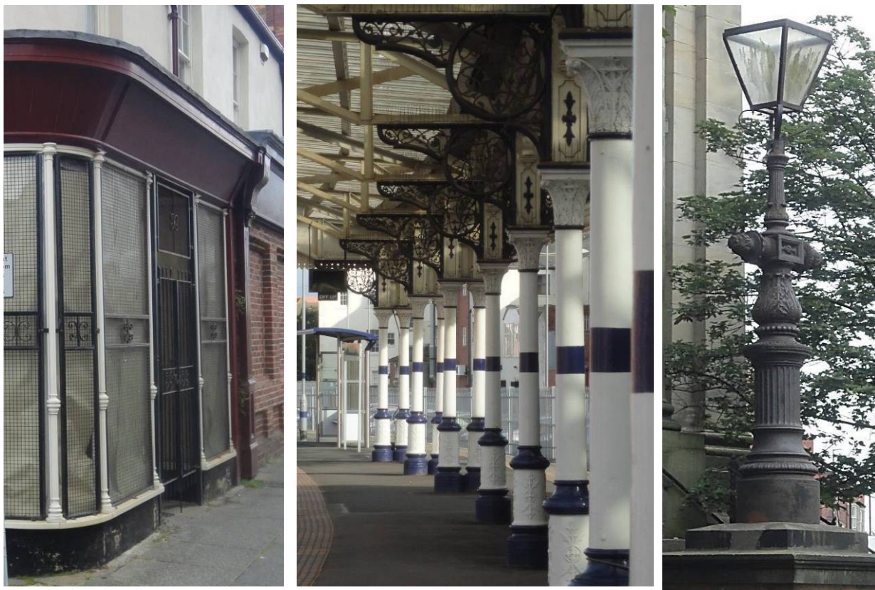
Fig 33. 9 Whitby Street with colonettes and traditional iron shop gate.
