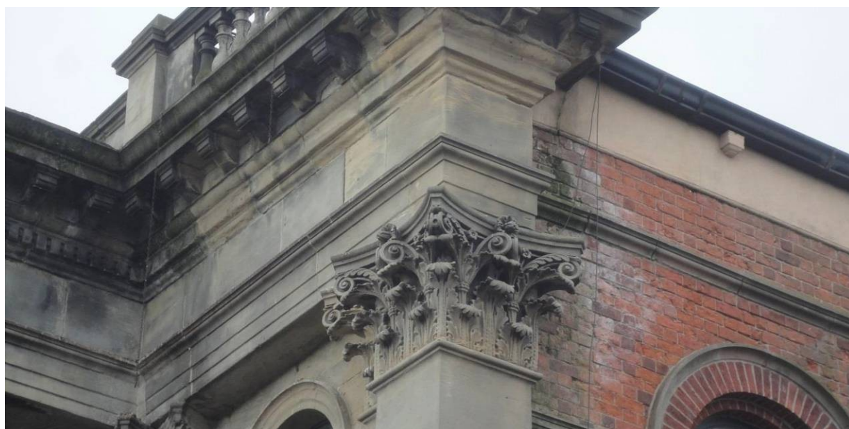
Fig 31. The finely detailed, classical ashlar front of the Wesley Methodist Church.
