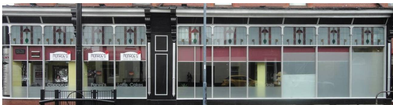
Fig 28. Shopfront at 31-32 Church Street, Hillcarter Hotel.
