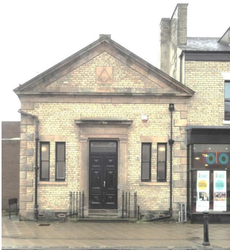
Fig 6. Masonic Lodge, Upper Church Street.
