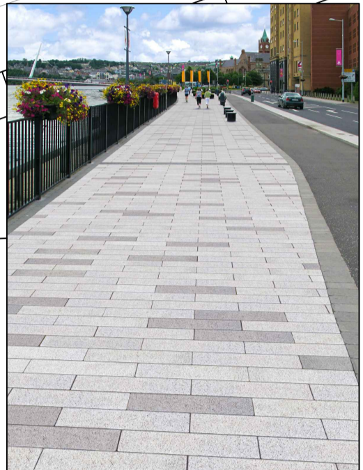
Manhattan PCC granite finish blocks (600x150x80mm); 75% silver - 25% mid grey (Tobermore or equal approved)
