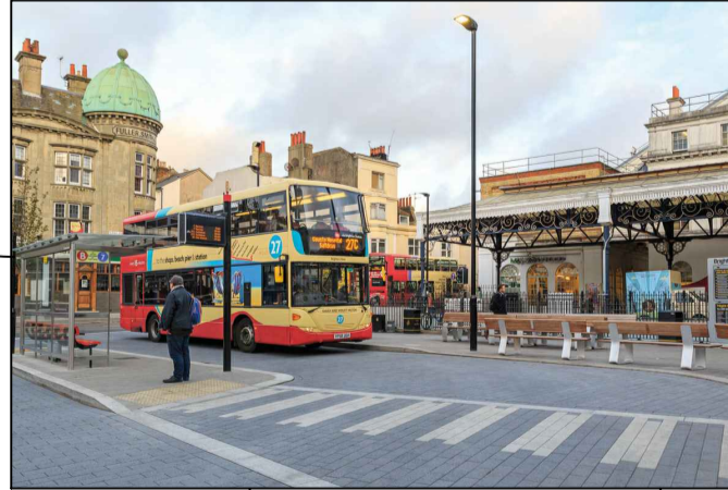
City-pave Vs5 granite aggregate blocks (150x100x100mm); dark grey & sandstone to crossing (Tobermore or equal approved)
