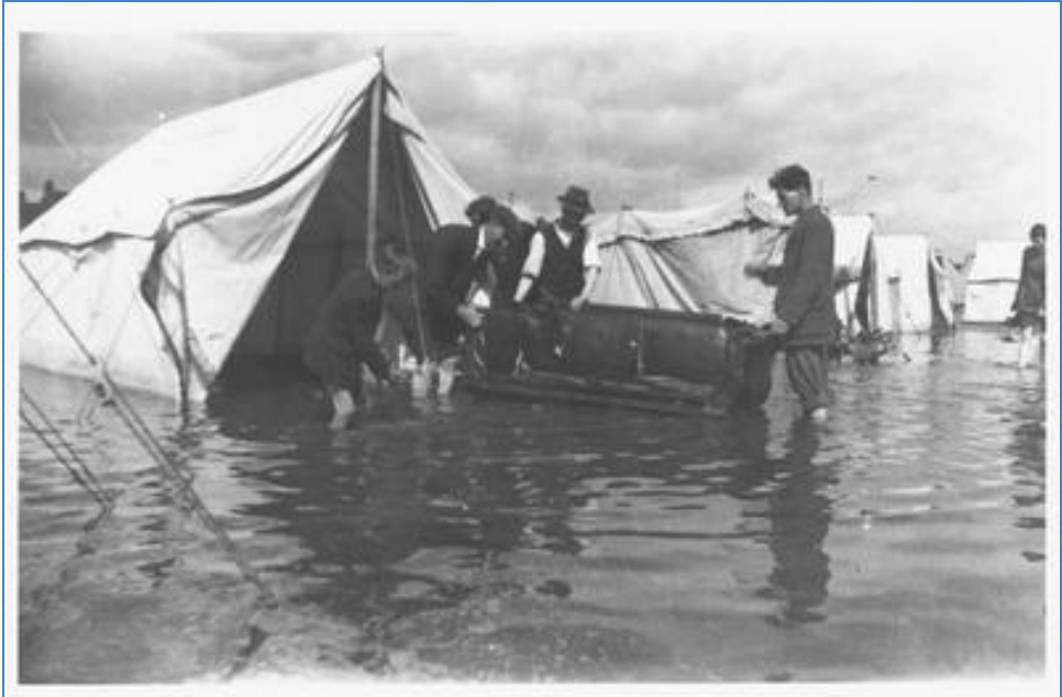
Figure 3 - Seaton Carew flooding in 1922
