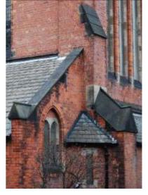
Joseph's Church and Nos. 26-28 Victoria Road. Pointing – the way that mortar (traditionally lime-based) is finished off – is generally flush or slightly recessed. The roughness of older bricks tends to make pointing more visually prominent, whilst the crisp lines of the rubbing brickwork is meant to make pointing less noticeable.
