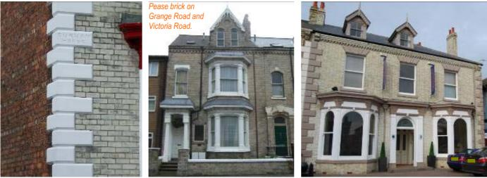
Bricks are predominantly laid in simple stretcher bond on front elevations, with English garden wall bond used mainly on side and rear elevations, with either 3 or 5 rows of stretchers to 1 of headers. Examples of Flemish bond (alternate headers and stretchers in every course, with headers placed centrally between the stretcher immediately above and below) are a rare stylish flourish, seemingly only found at St
