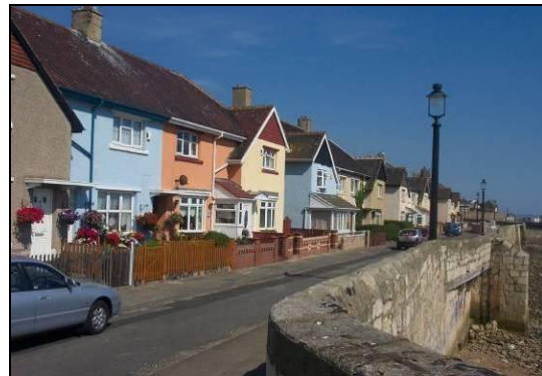
Town Wall east
