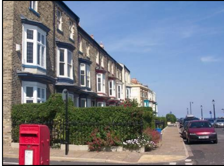
Strong edge at Albion Terrace
