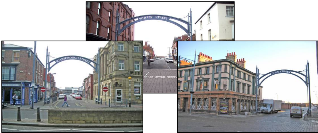
Figure 4.7: Photographs illustrating the lack of containment
