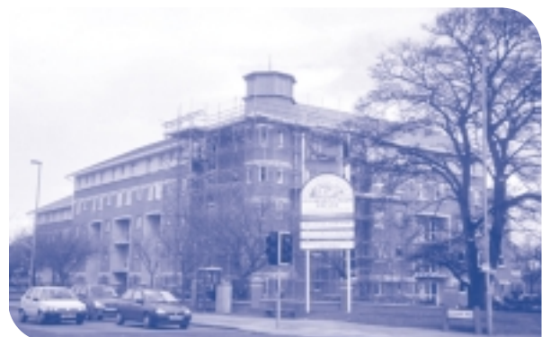
Photograph 6.3: Retirement Home, Linthorpe Road, Middlesbrough
