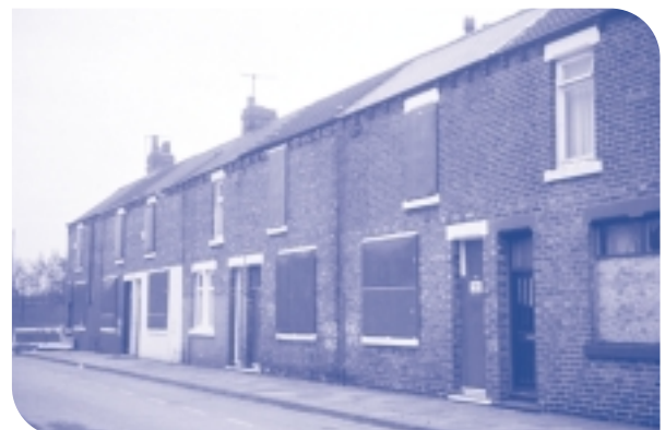
Photograph 6.1: Housing Demolitions / Low Demand Housing
