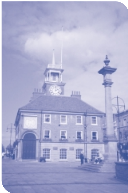
Photograph 3.2: Stockton Town Hall
