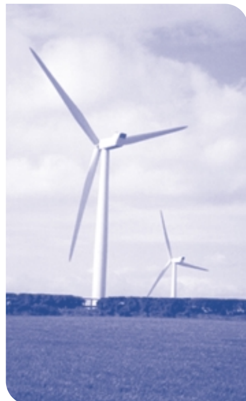
Photograph 10.1: Wind Turbines, Hartlepool
