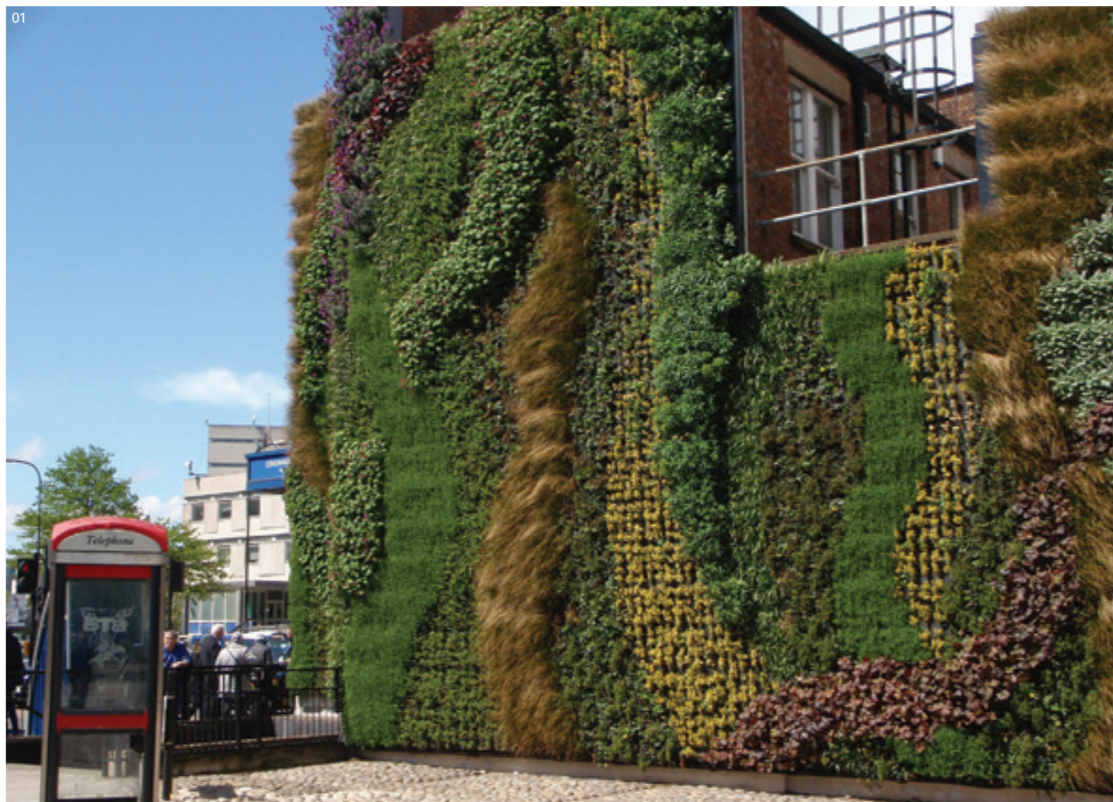
01 Edgware Road green wall, London, Transport for London
