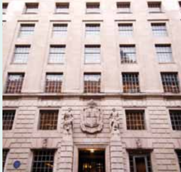
The Department of Energy and Climate Change expects to cut energy bills
