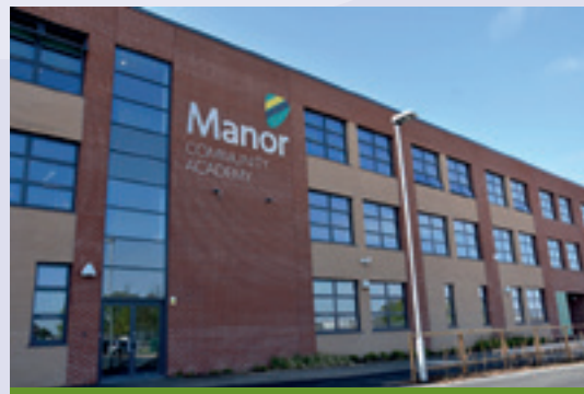
Manor Community Academy opened a brand new building, sponsored by Northern Education Trust.
