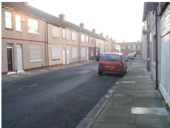
Image 1 – Terraced Housing in Mildred Street
