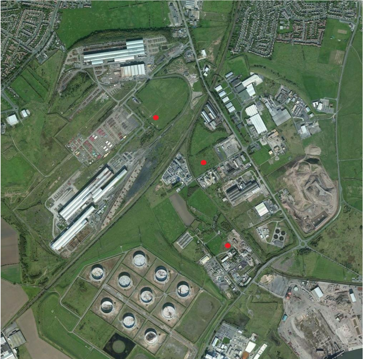
Figure 6: Aerial photograph of site Proposed turbine positions are indicated by red dots.
