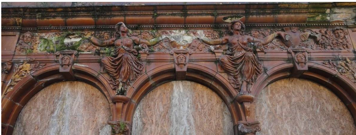
Fig 43. Faience arcade at The Shades, showing critical condition.
