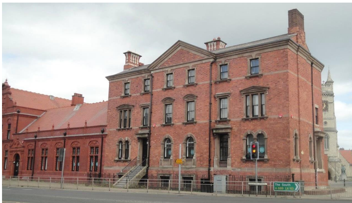
Fig 69. Former Police Station (right) and Library (left), now occupied by CCAD.
