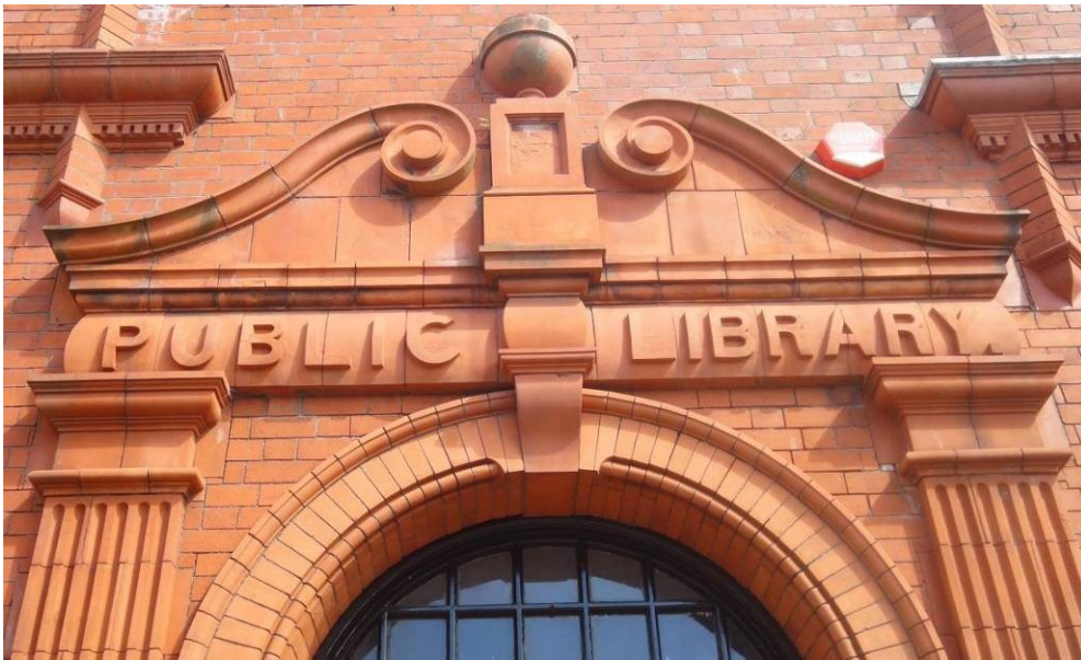
Fig 29. Normanby brick from Middlesbrough at the Public Library, now CCAD.
