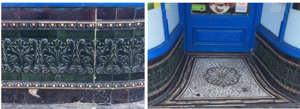
Figs 36 and 37. Tiled stallriser and mosaic pavement at 13 Church Square.
