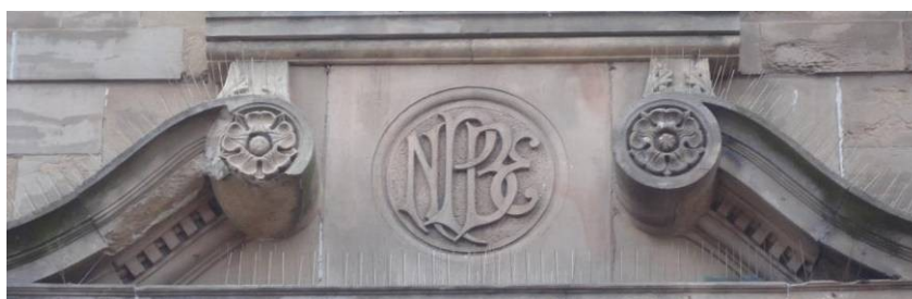
Fig 52. Doorpiece monogram at former National Provincial Bank, Church Street.
