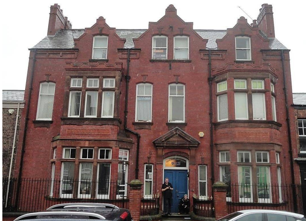
Fig 73. West Hartlepool Club, 9-13 Scarborough Street.
