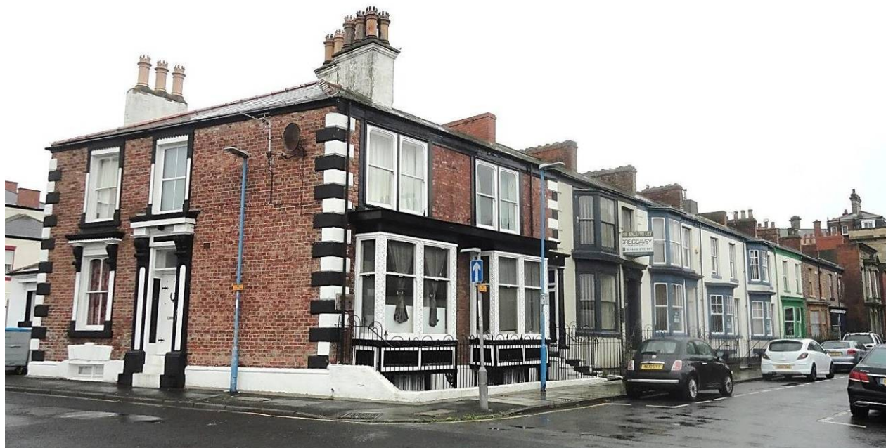
Fig 72. 36 Exeter Street to left and Scarborough Street extending to right.
