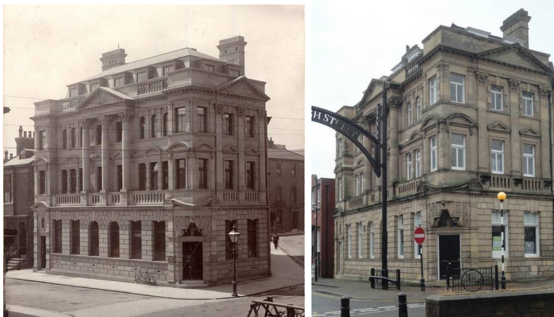
Figs 53 and 54. 38 Church Street, former York City and County Bank.
