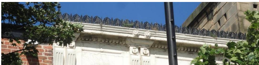
Fig 41. Classical brattishing crowning the ornate wallhead at 70 Church Street.
