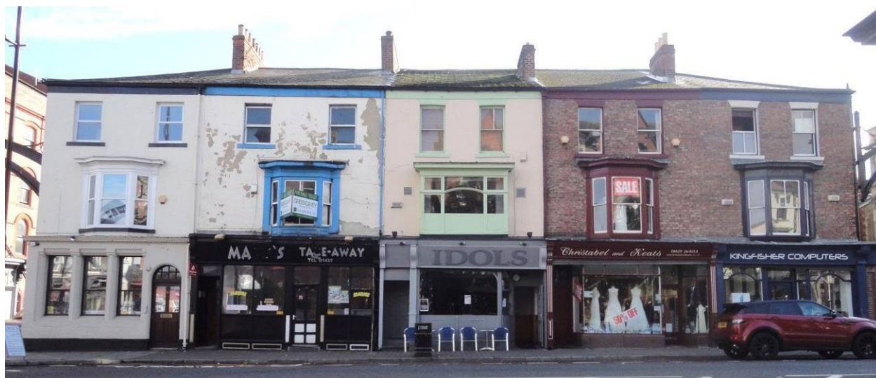
Fig 22. Symmetrical and traditionally detailed Nos 33-37 Church Street introduce the broad avenue to the south-east with the street's typical combination of shopfronts, canted and box windows and paired windows.
