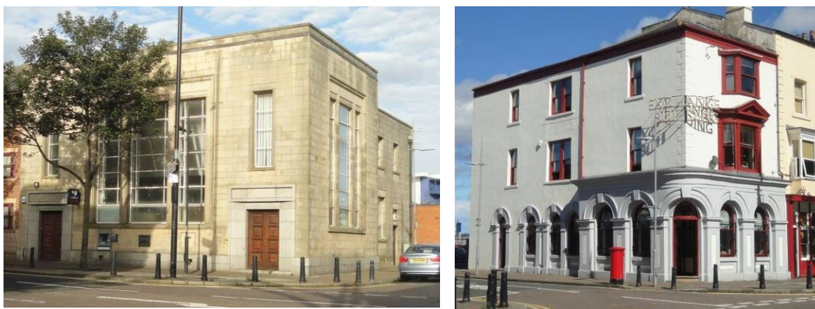
Fig 55. 65 Church Street, former Yorkshire Bank.
