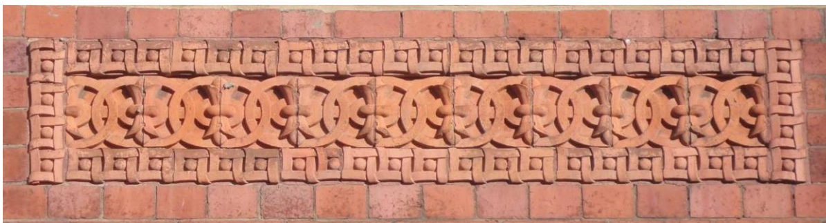
Fig 79. Detail of ornamental brickwork, former West Hartlepool Club, Scarborough Street.
