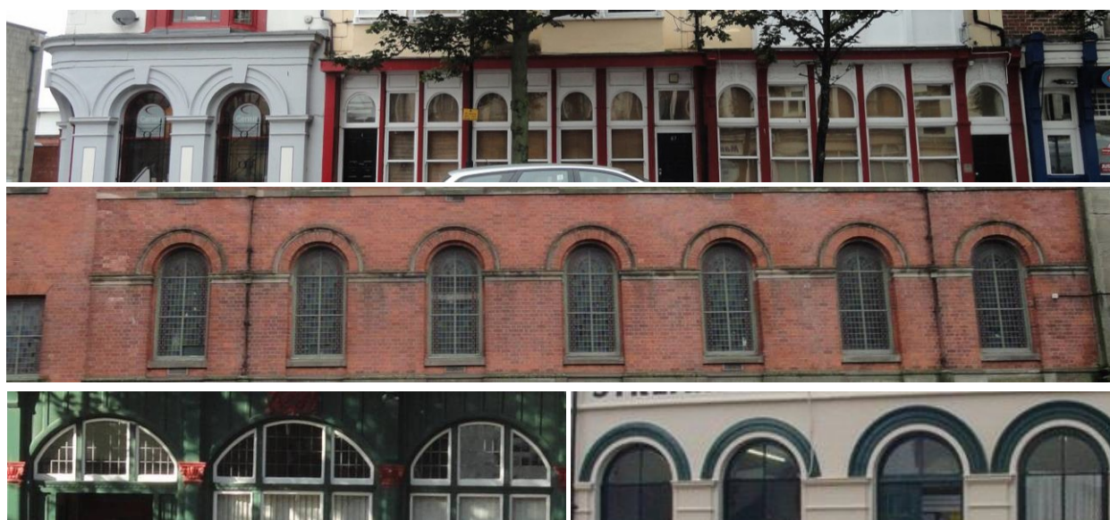
Fig 42. Examples of the arcade theme that runs through the conservation area.
