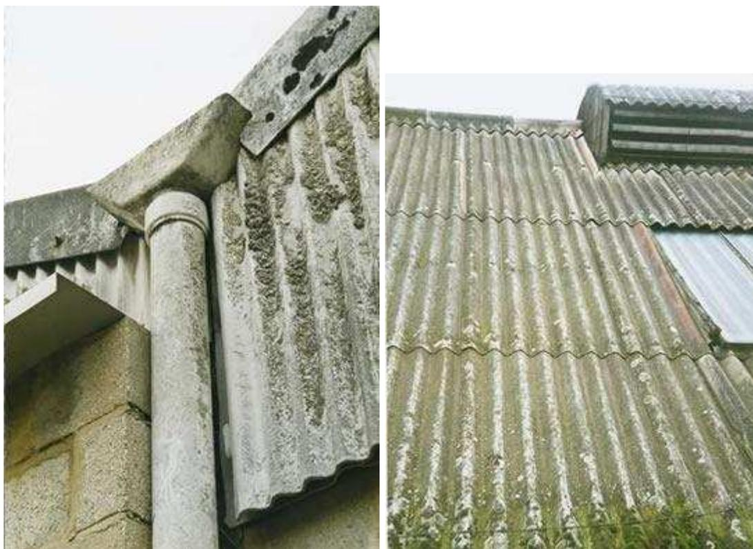
Asbestos cement is a mixture of asbestos (usually about 10-15% of the total product) and cement. It is often seen as corrugated roofing panels on sheds, farms and industrial buildings, but can also be used to make drain pipes, flues and water tanks. It is usually grey/white in colour, hard and inflexible.
