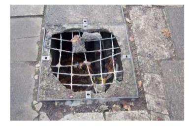
A rigid footway, with a damaged `13<sup>-</sup>1' inspection chamber cover.
