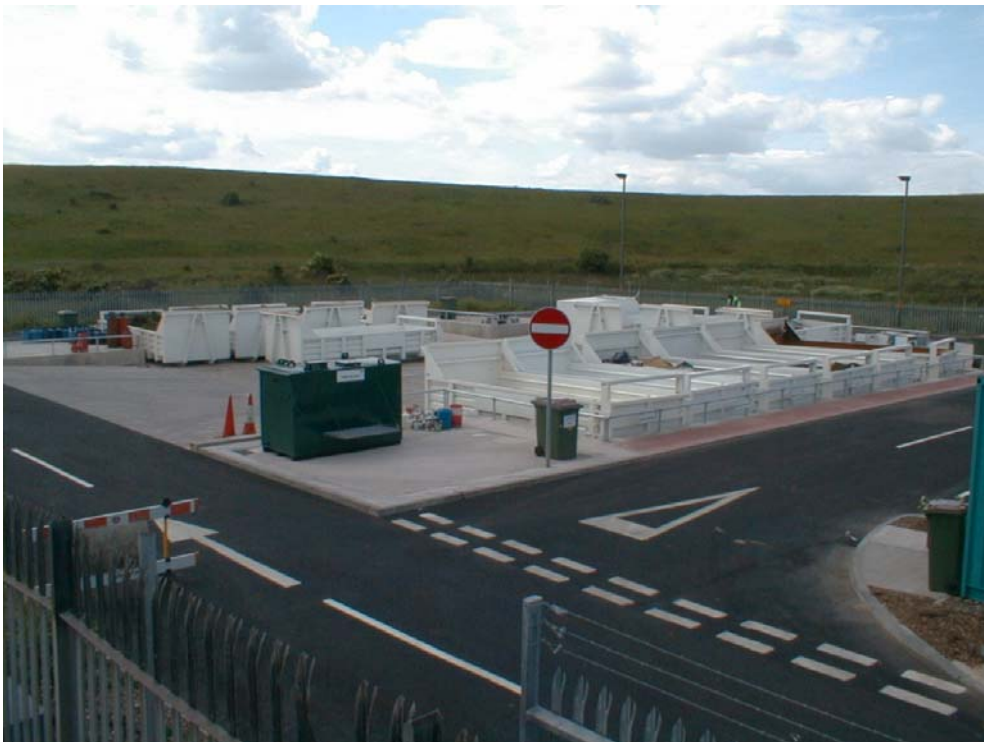
Figure 3.3 Household Waste Recycling Centre
