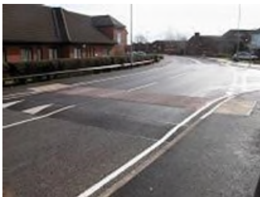
New Carriageway Surface
