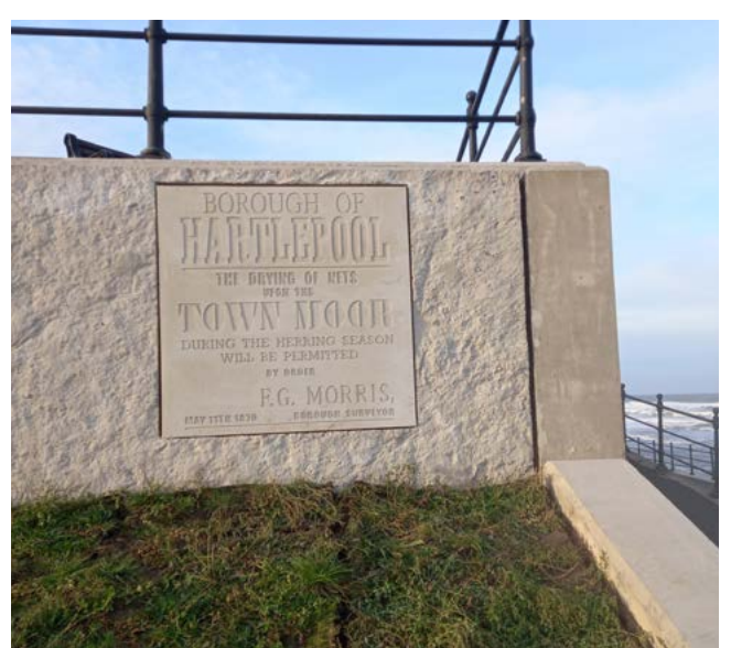
One of the plaques built into the rear retaining wall
