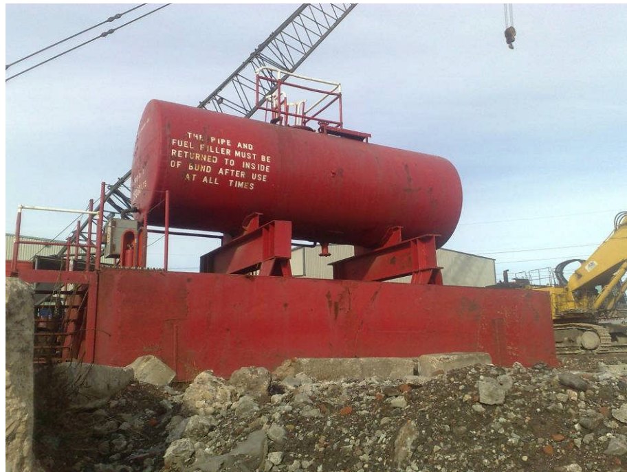
Plate 1: Tank 1 - Main bulk diesel storage tank
