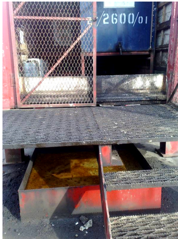
Plate 9: Additional spill containment below oil storage area.
