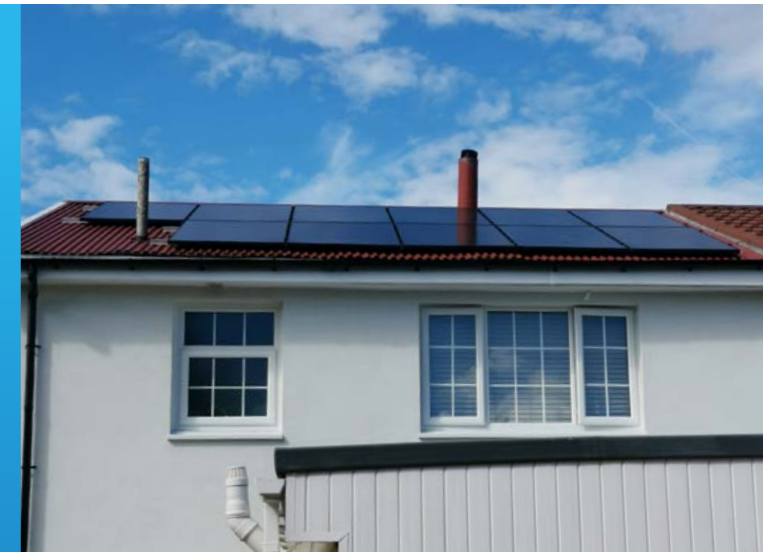
Solar panels fitted to the family home
