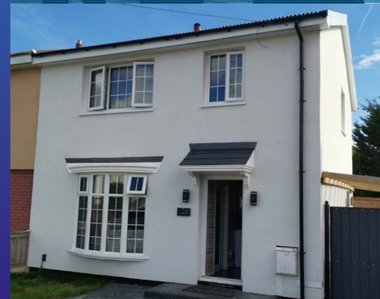
Family home after the installation of external solid wall insulation
