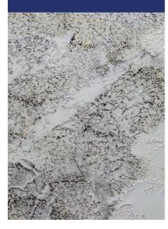
During the colder months condensation becomes a major problem in many British homes. It is caused when warm, moist air hits a cold surface such as a window or external wall and condenses, running down the cold surface as water droplets. If left this can develop into black mould which looks and smells bad and can cause health problems as well as thousands of pounds worth of damage to clothes, furniture, books, shoes and decorations.
