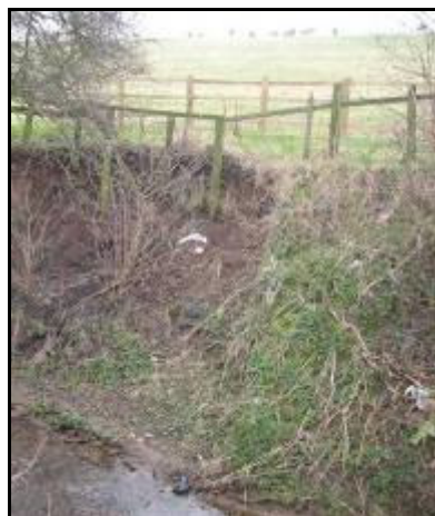
Figure 2.5 Large bank failure on right hand bank facing downstream
