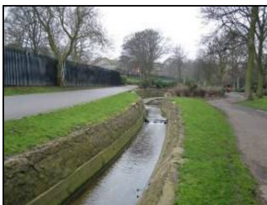
Figure 2.3 Reprofiled vertical banks, widened and deepened channel and uniform flow conditions upstream of the park
