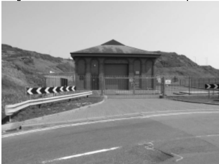
Figure 4: Saltburn Northumbrian Water Treatment Works grid reference NZ ???
