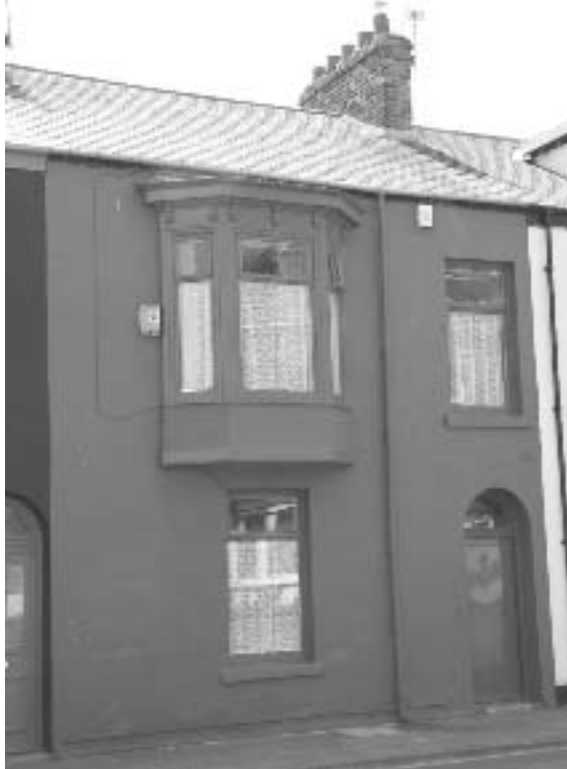
Example 4 - Headland Conservation Area. Ground and first floor replacement windows
