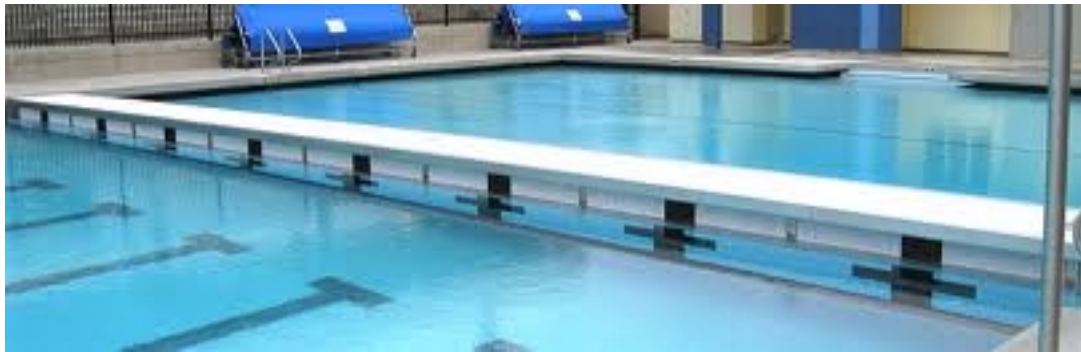
Diagram 1 – Example of typical pool bulkhead installation
