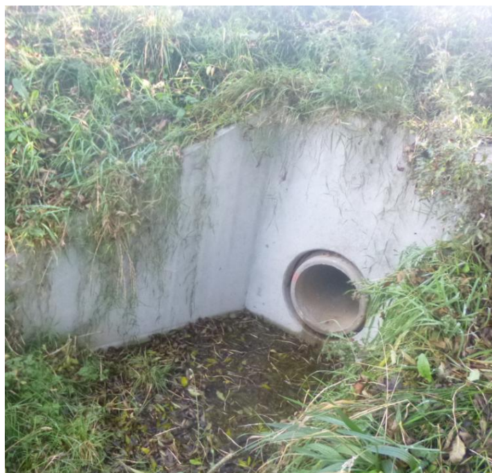
Fig 2 New Headwall protecting North Close.
