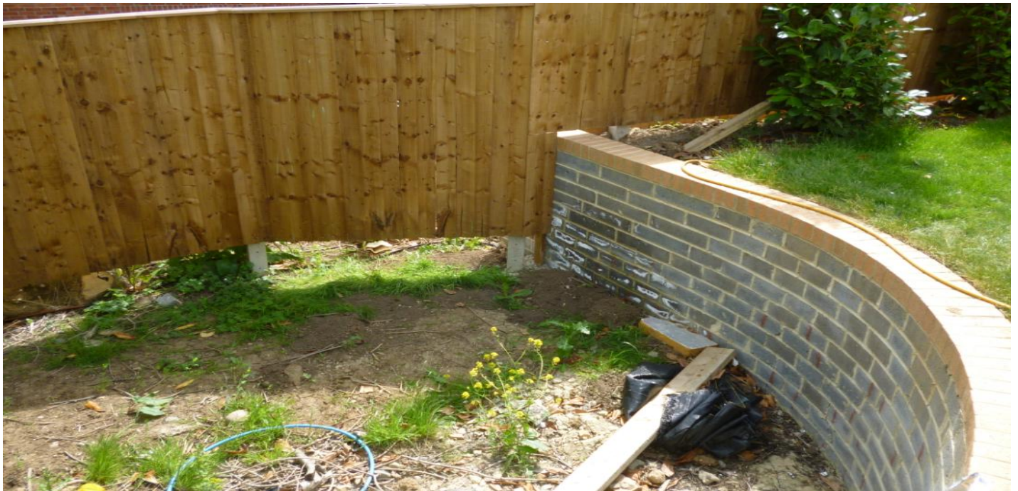
4) view to 'curved' retaining wall section (approx. 1.1m lower than raised garden level)
