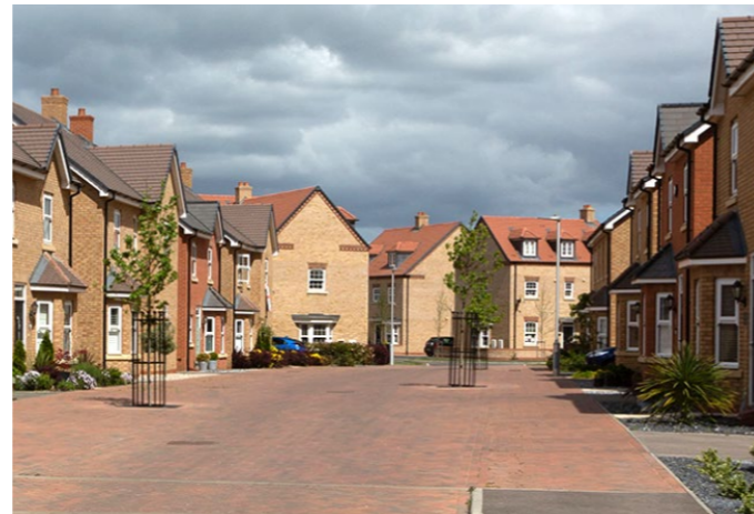
Example shared surface Lane with planting.
