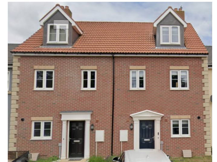
Meter box impacting on elevation
