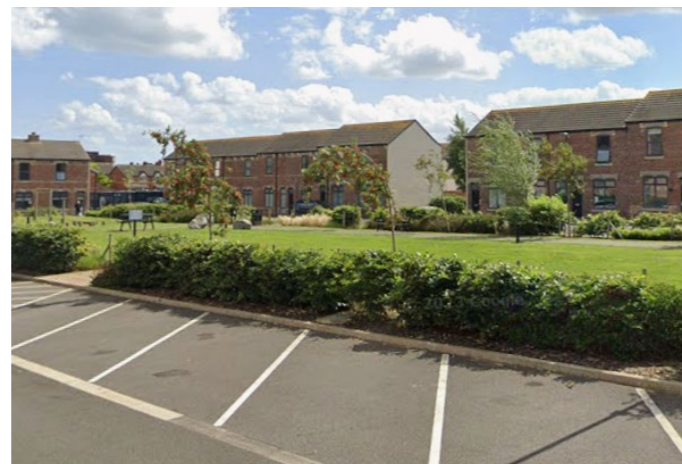
Courtyard Parking - Hatlepool
