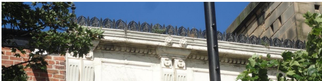
Fig 39. Classical brattishing crowning the ornate wallhead at 70 Church Street.
