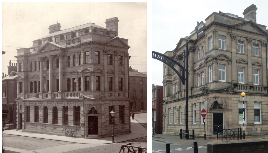
Figs 51 and 52. 38 Church Street, former York City and County Bank.
