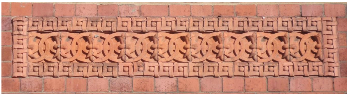
Fig 77. Detail of ornamental brickwork, former West Hartlepool Club, Scarborough Street.
