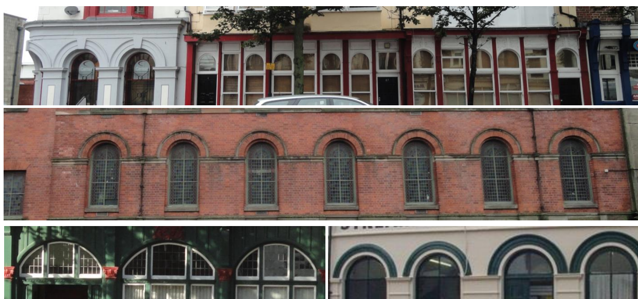
Fig 40. Examples of the arcade theme that runs through the conservation area.
