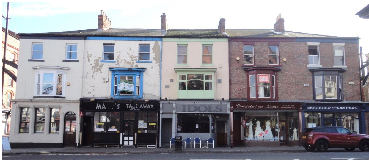
Fig 22. Symmetrical and traditionally detailed Nos 33-37 Church Street introduce the broad avenue to the south-east with the street's typical combination of shopfronts, canted and box windows and paired windows.
