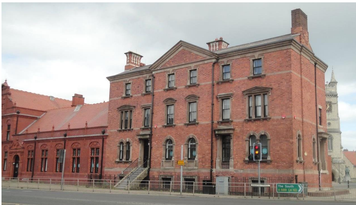
Fig 67. Former Police Station (right) and Library (left), now occupied by CCAD.
