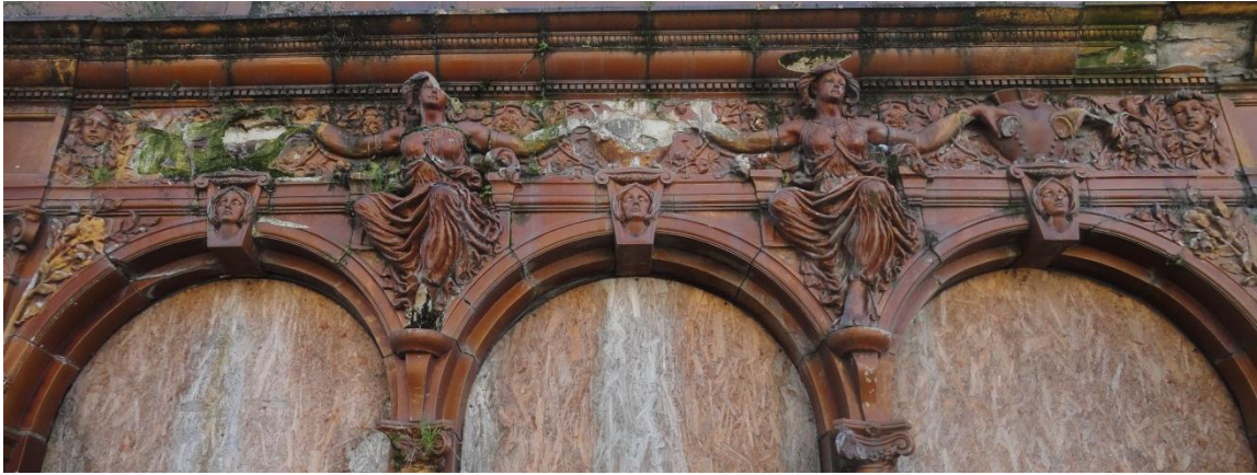
Fig 41. Faience arcade at The Shades, showing critical condition.
