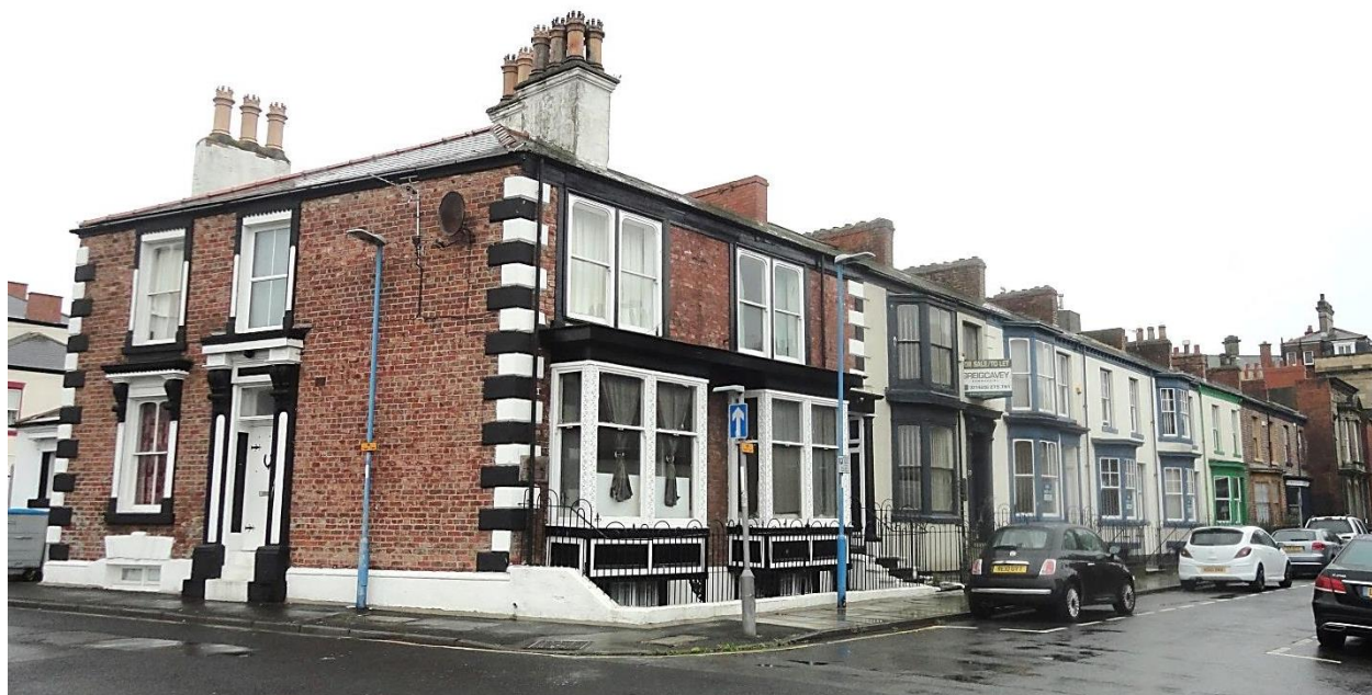
Fig 70. 36 Exeter Street to left and Scarborough Street extending to right.
