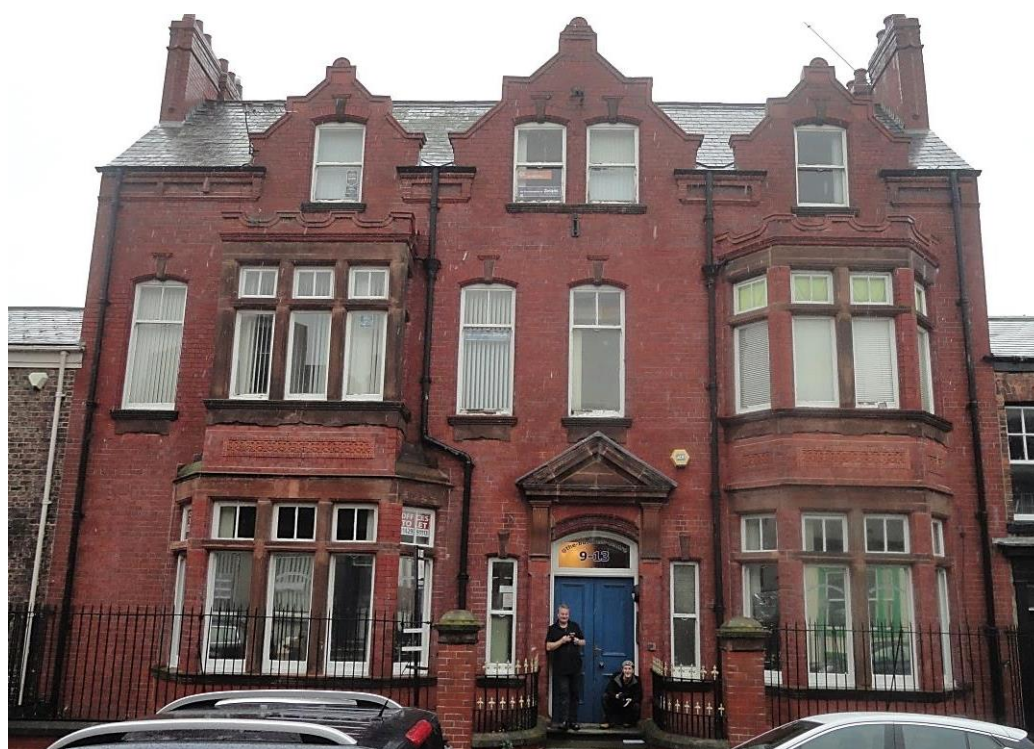
Fig 71. West Hartlepool Club, 9-13 Scarborough Street.
