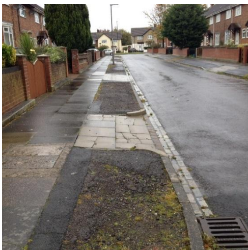
Existing damaged surfacing shown above.
