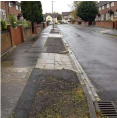
Existing damaged surfacing shown above.
