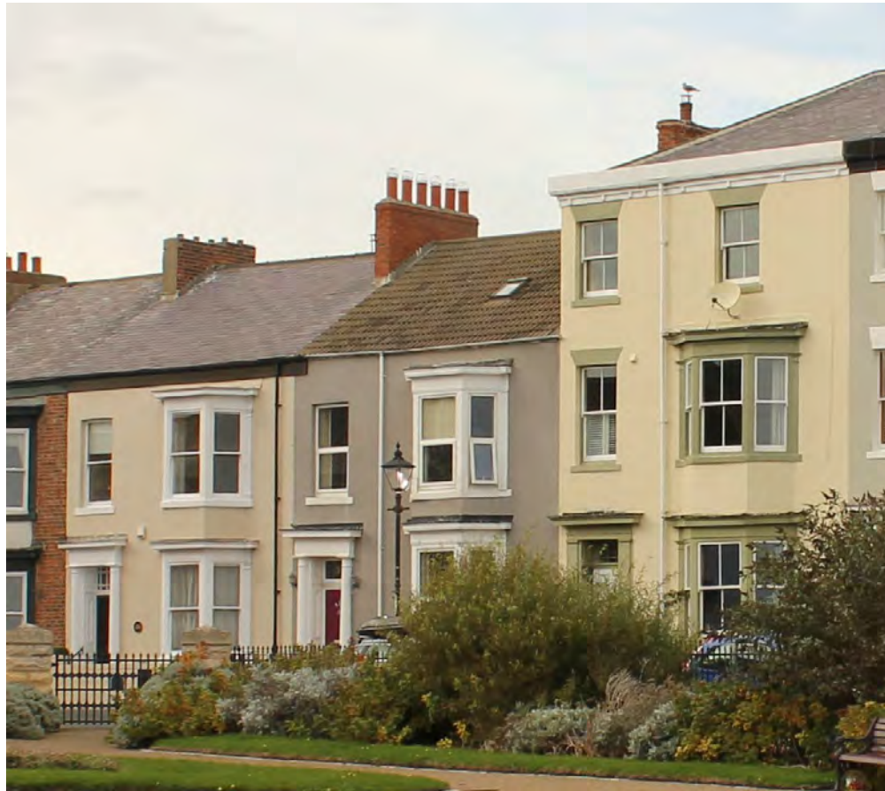
Modern concrete tile is not an acceptable material on historic buildings in the conservation area
