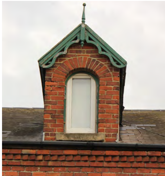
The character of the dormer on the right has been severely impacted by an inappropriate uPVC replacement window which makes no attempt to reproduce the historic form shown on the left
