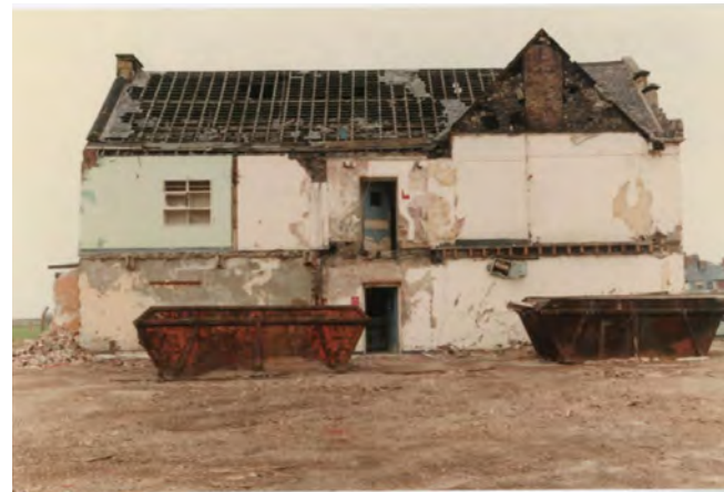
The Friarage Manor House during demolition in 1987
