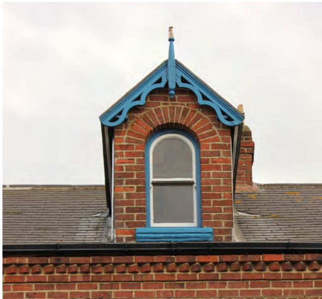
The character of the dormer on the right has been severely impacted by an inappropriate uPVC replacement window which makes no attempt to reproduce the historic form shown on the left
