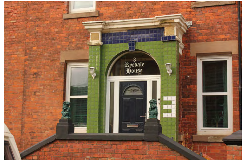
Imposing individuality on this porch in Beaconsfield Street has both impacted on the building's appearance and likely causing damaged to historic fabric below the modern tiling
