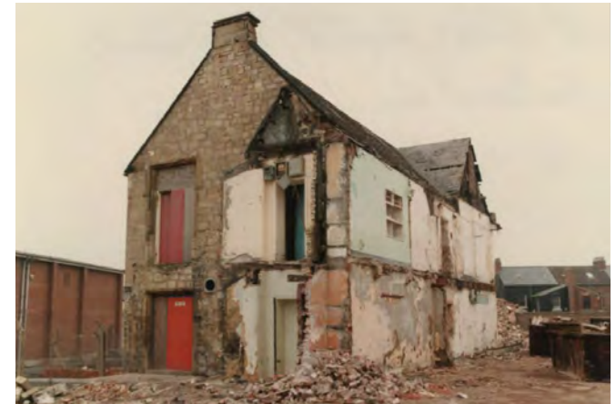
The east elevation. Note the cement render below the west elevation where the basement windows were once positioned
