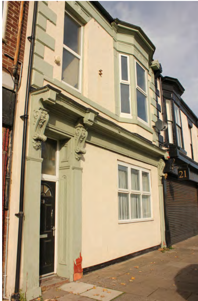
Former shop on Northgate which retains a number of decorative features including console brackets and fascia.
