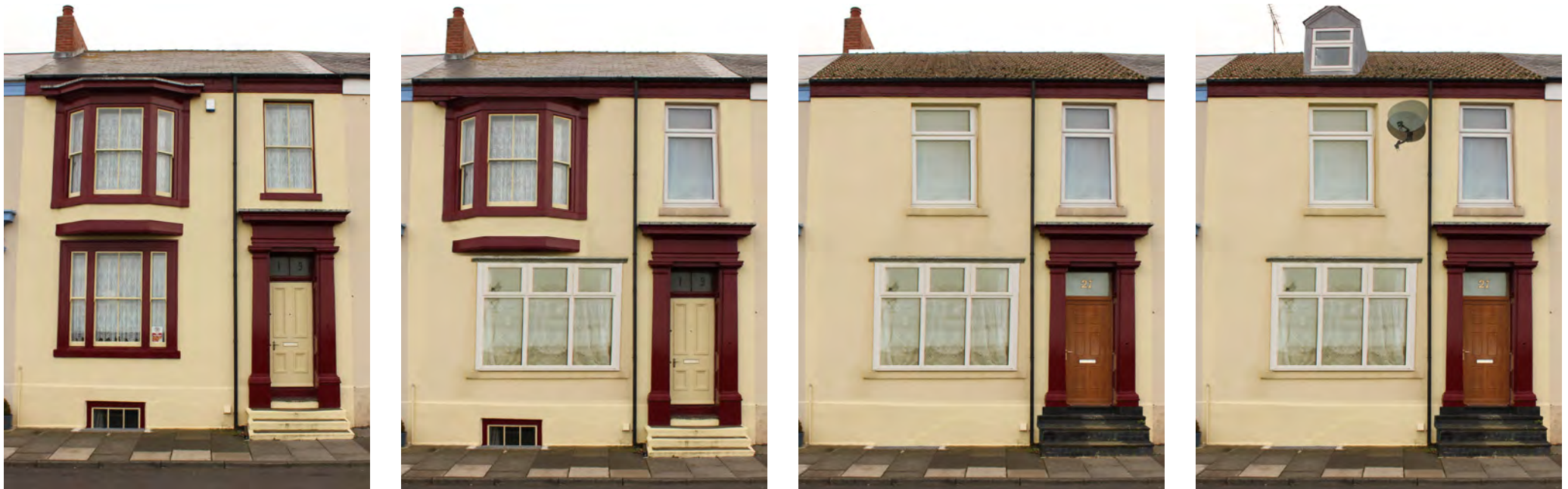
A manipulated image showing how cumulative alterations and loss of original features can be damaging to a property
