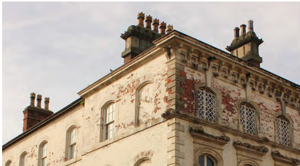
Substantial chimneys on Southgate
