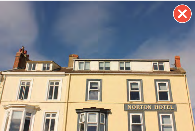
Inappropriate dormers on historic buildings
