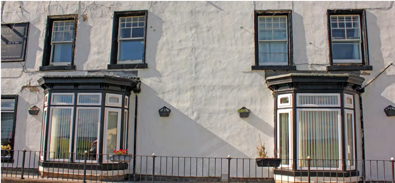
These bay windows have been replaced with uPVC. Their frames are much wider and heavier looking than the historic windows on the first floor.
