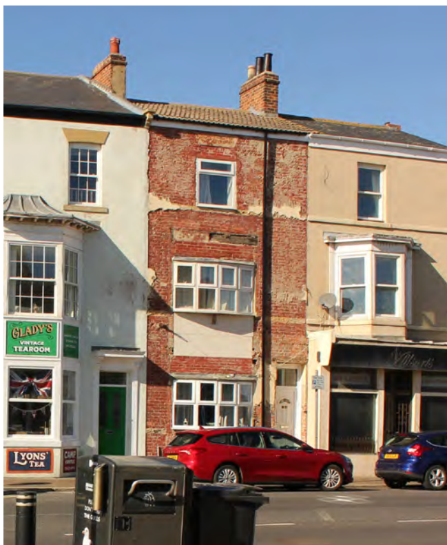
Not only has the render been removed from this terrace, but it has also suffered from the loss of traditional windows replaced with inappropriate modern bow-bays on the ground and first floor. The second floor opening has been reduced in height.
