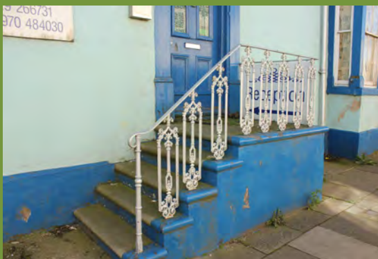
Historic railings on Church Street
