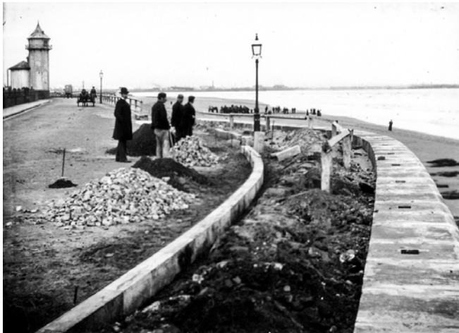
Construction of Seaton Promenade (Hartlepool Museum Service)
