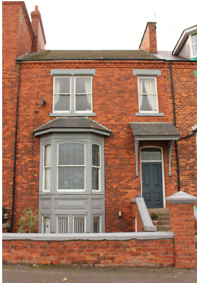
This manipulated image shows the impact on the appearance of this residence of removing historic windows and installing uPVC windows
