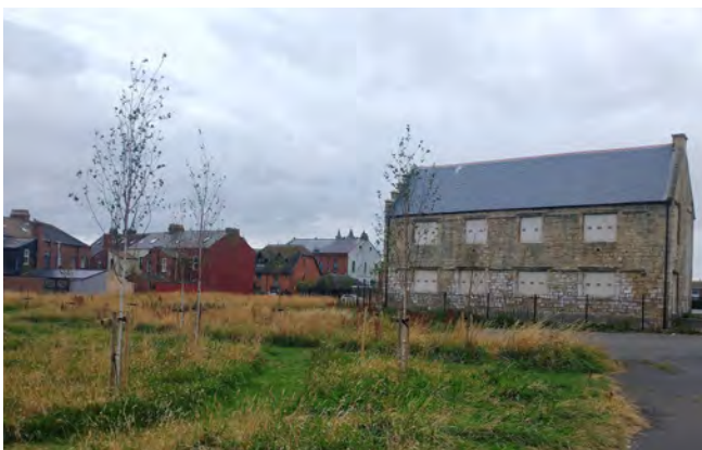
The Friarage Building
