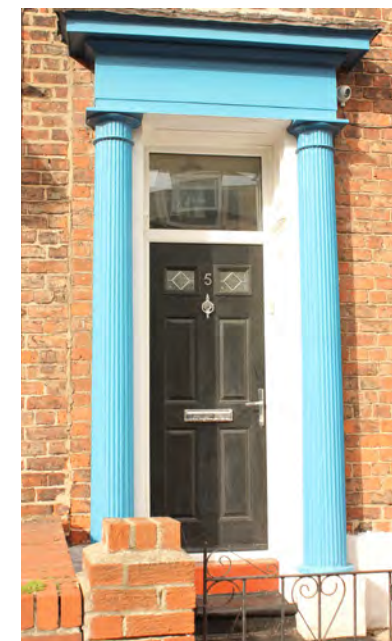
A modern composite door incorporating glazing and modern chrome fittings is not appropriate.
