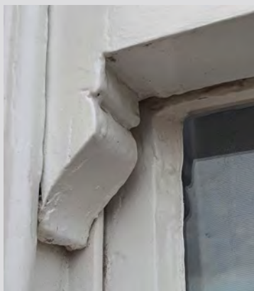
A typical late 19th century window horn
