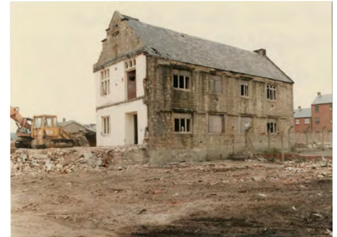
The east elevation. Note the cement render below the west elevation where the basement windows were once positioned
