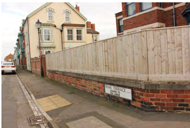
Inappropriate close-boarded fence facing a street
