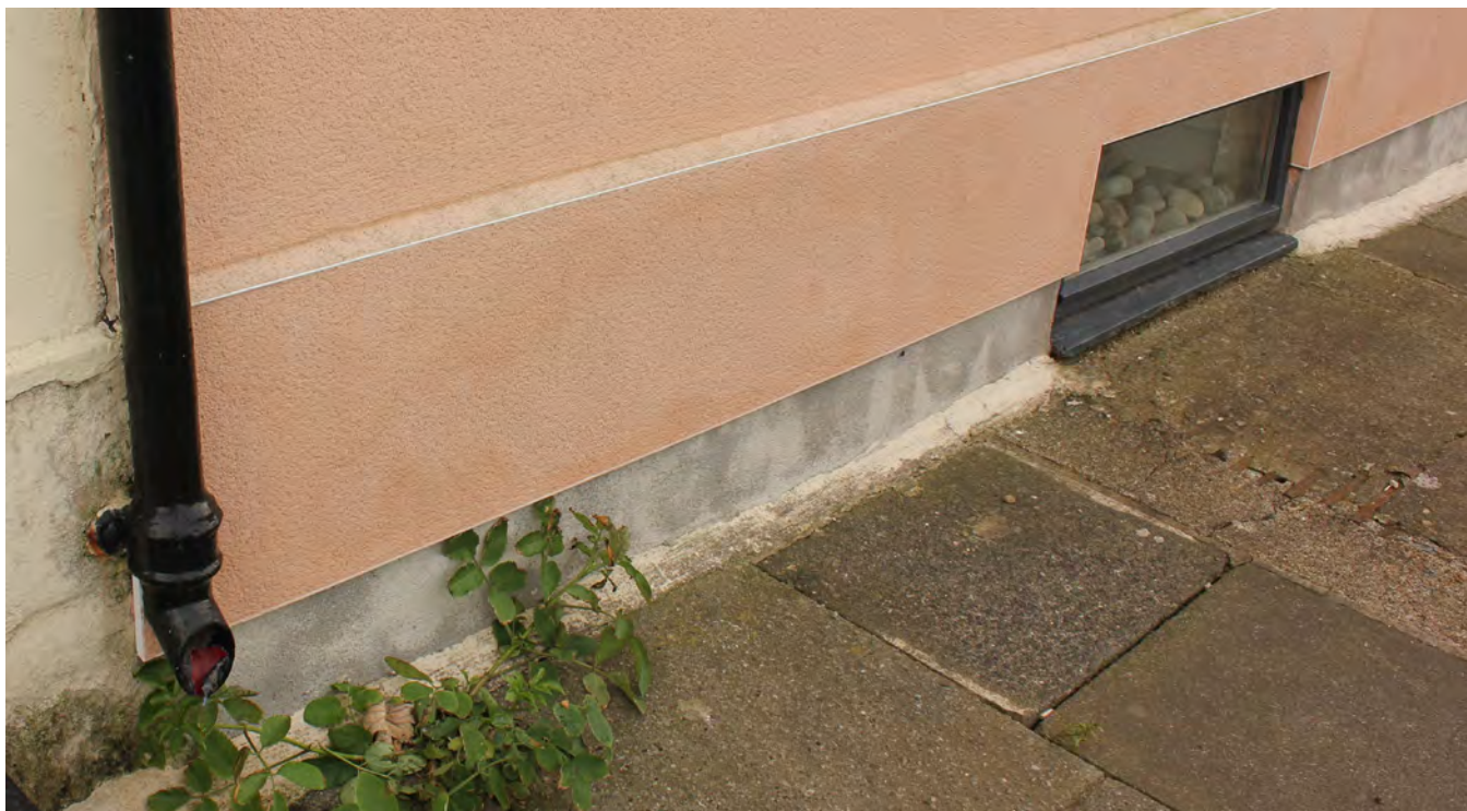
This modern render is raised above the finish on the adjacent building and has a distinctive plastic edging strip. If utilising a modern impermeable material, it may be causing more harm than good on this historic building.
