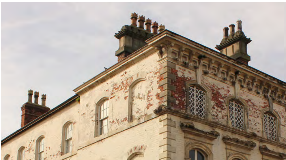
Substantial chimneys on Southgate
