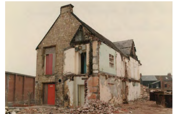
The east elevation. Note the cement render below the west elevation where the basement windows were once positioned
