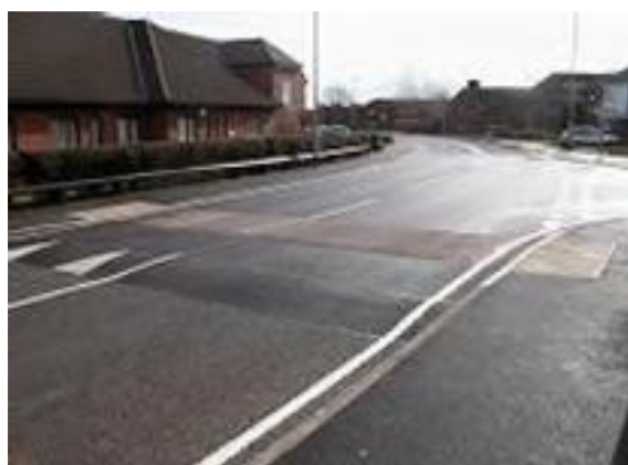
New Carriageway Surface
