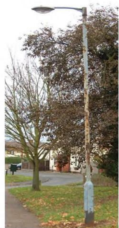
Steel street lighting column in poor condition.
