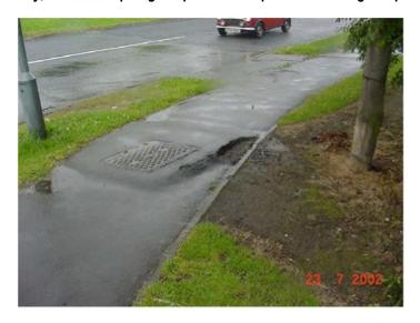
$\frac{\text{ls urgent treatment required?}}{\text{The defect is measured at 40mm and is therefore considered a Safety Hazard.}}$
