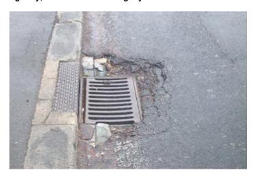
$\frac{\text{Is urgent treatment required?}}{\text{The defect is measured at approximately 50}} - 75 \text{ mm, which is above the intervention level, and is therefore considered a Safety Hazard.}}$
