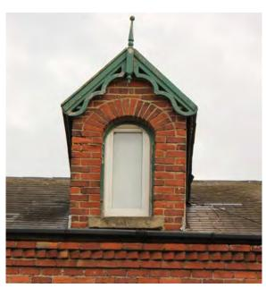
The character of the dormer on the right has been severely impacted by an inappropriate uPVC replacement window which makes no attempt to reproduce the historic form shown on the left
