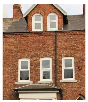
An example of inappropriate uPVC windows; the frames are too heavy, their standard shape fails to respond to the arched window openings and make a poor attempt to imitate sashes.
