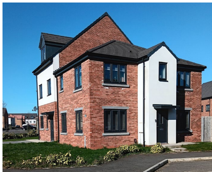
Corner turning building - Seaton Meadows
